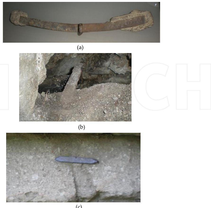
**Figure 4.** Variations in iron clamps used in historical stone masonry walls
