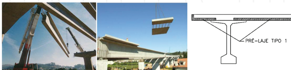
Figure 8. Placement of precast beams and pre-slabs.
