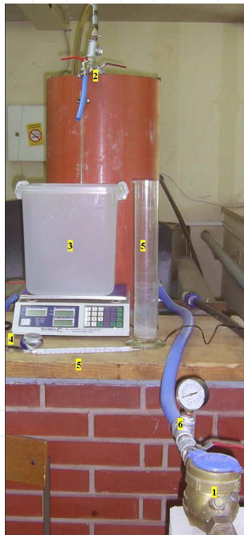
Figure 3. Part of the water supply pipeline downstream from the water meter (1) in the Hydraulic Laboratory of the Faculty of Civil Engineering in Subotica. 2 - stop valve, 3 - vessel with scale for measuring water quantity flown through the water meter, 4 - stop-watch, 5 - measuring cylinder and thermometer, 6 - manometer.
