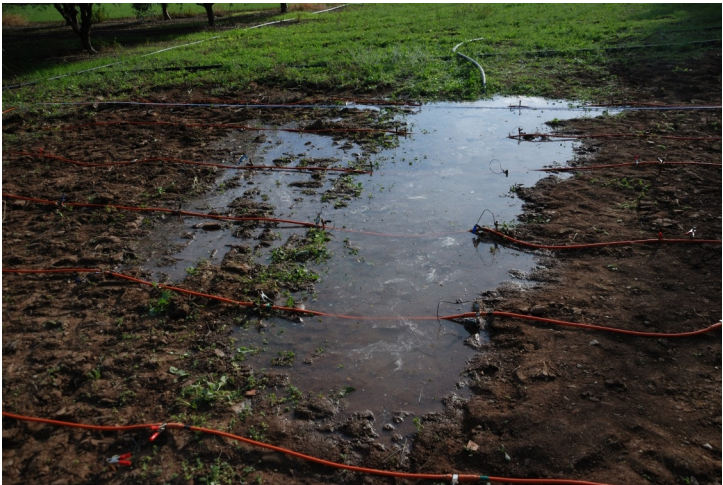
Figure 2. Leakage as observed from the surface
