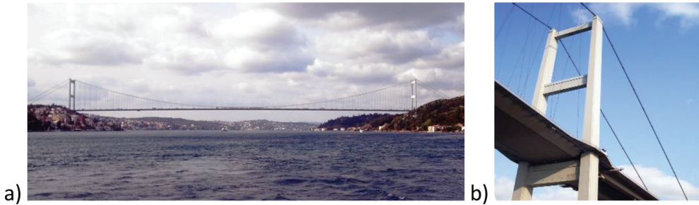
Figure 21. First Bosphorus Bridge: (a) side view; (b) tower and aerodynamic low profile deck.
