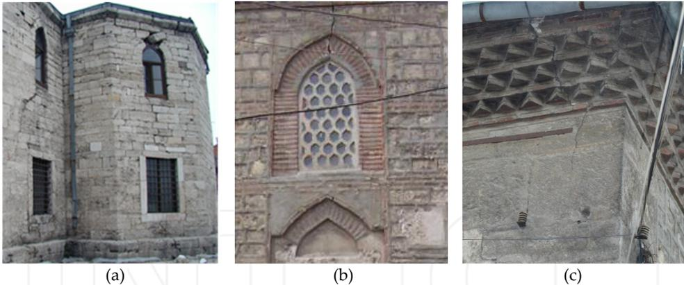
**Figure 10.** a) cracks developed in the walls and above windows of Kadi; and b, c) damage in in the walls of Sarachane mosque
