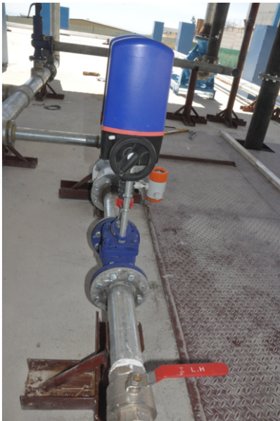
Figure 9. Analog valve (left) and pressure relief valve (right)
