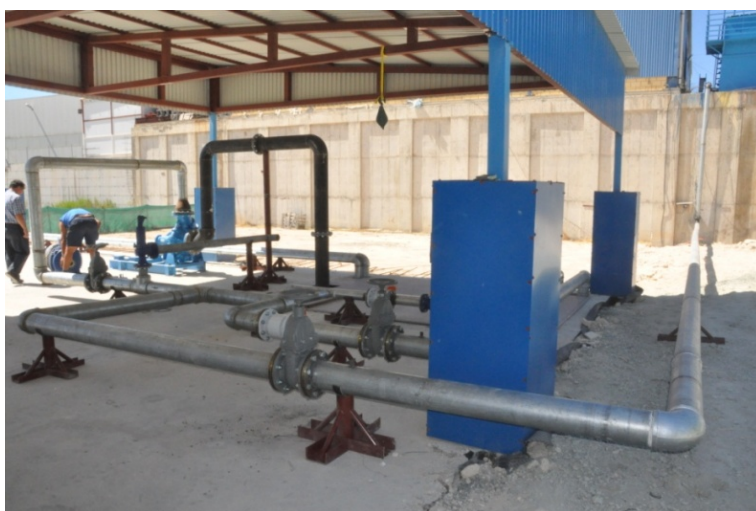
Figure 7. Photo of a part of the pipe network as it has been constructed
