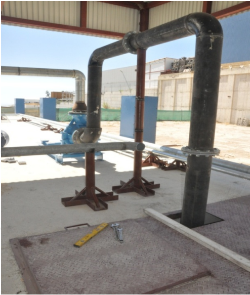
Figure 8. Pipe network during construction
